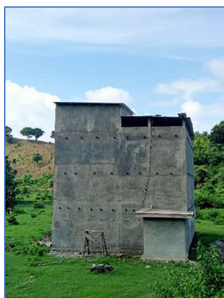
Figure 1. Edible house at research site
