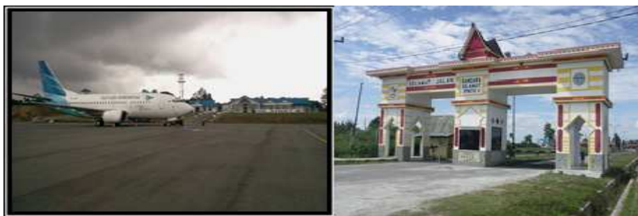
FIGURE 1 SILANGIT AIRPORT AND ROAD TO AIRPORT
